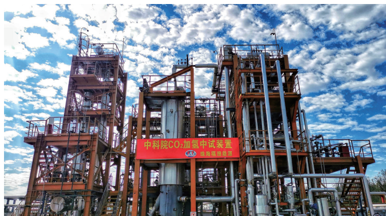
A Chinese pilot plant in Shandong province for producing 1000 tons/year of gasoline from carbon dioxide (CO 2 ) hydrogenation. (Image by HOU Shoufu)
