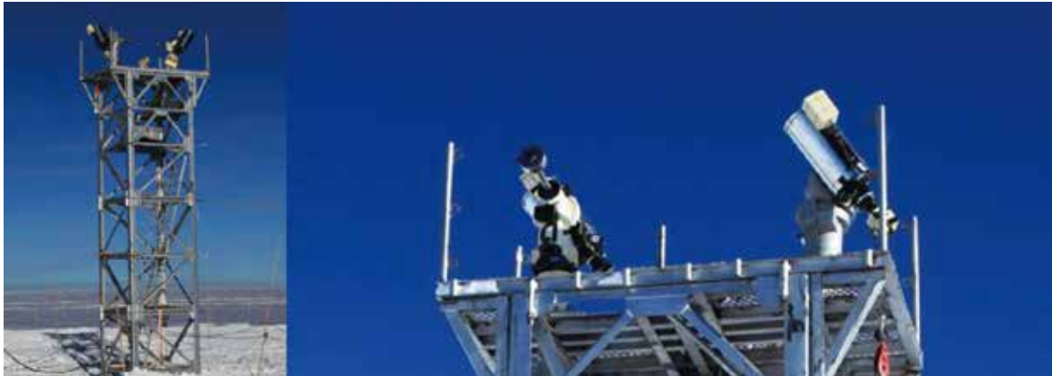
Figure 3: Two redundant KL-DIMMs and their eight-meter-high tower. (Credit: SHANG Zhaohui)
