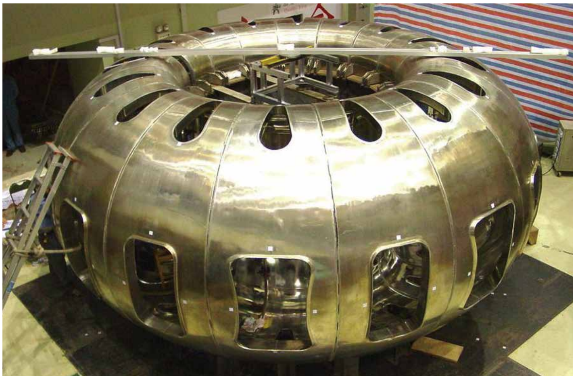
The vacuum vessel ring of EAST as seen in 2004, being installed. (Credit: CASHIPS)
