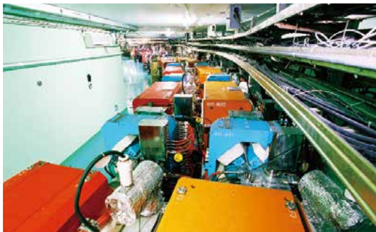
Inside the tunnel of BEPC when it was under upgradation (Image: IHEP)
