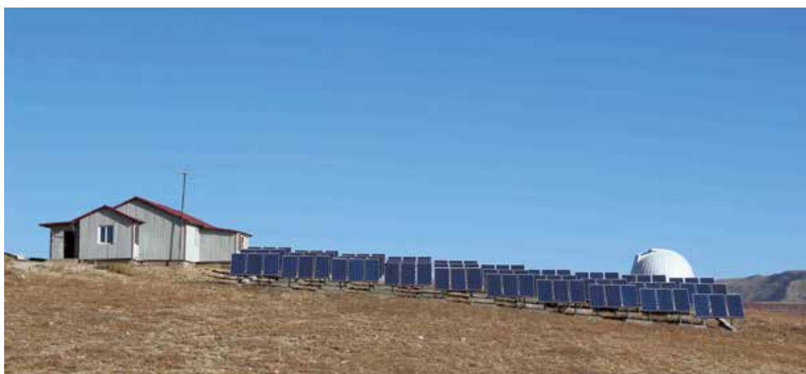
With joint efforts of NAOC and UBAI, a 20kW solar power station was launched at Maidanak Observatory for uninterrupted power supply of the 1-m telescope.
