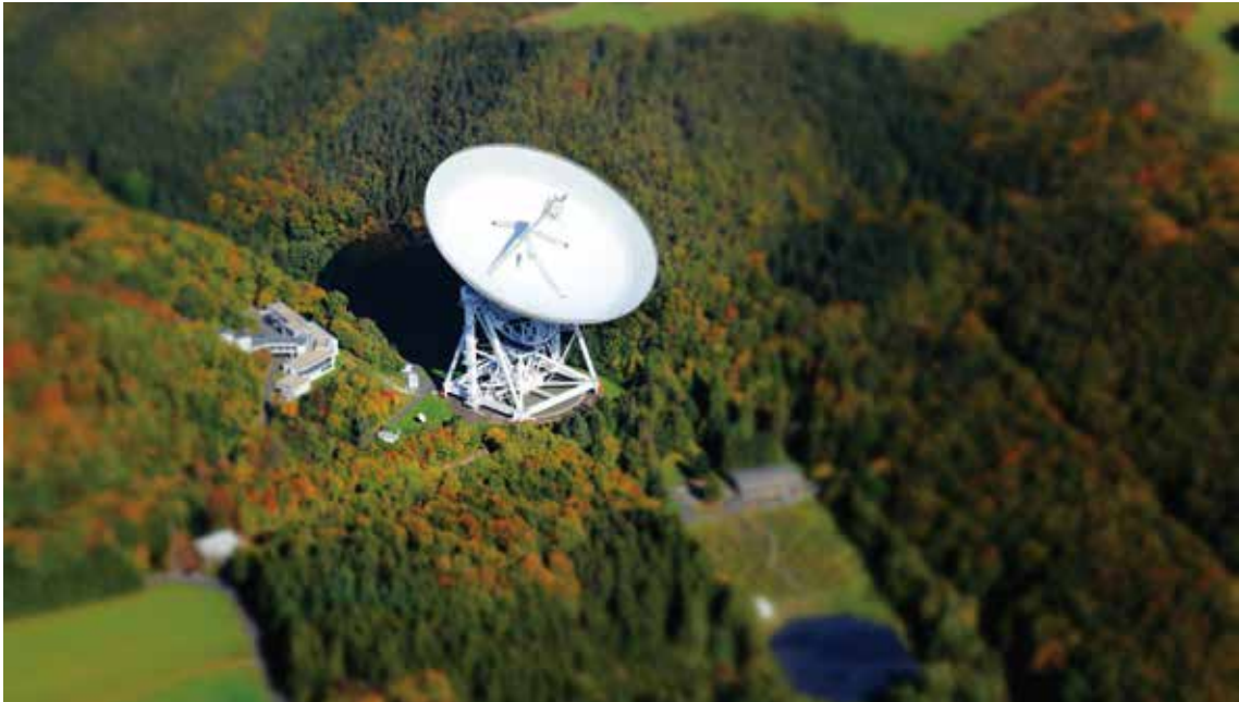
Aerial view of the Effelsberg Observatory near Bonn, Germany. Visible is the 100m Effelsberg telescope, the largest fully steerable telescope in Europe. Also visible are the low- and high-frequency antenna of the MPIfR's LOFAR station. Combined the observatory covers a frequency range from 10 MHz to 100 GHz. (Credit: MPIfR)
