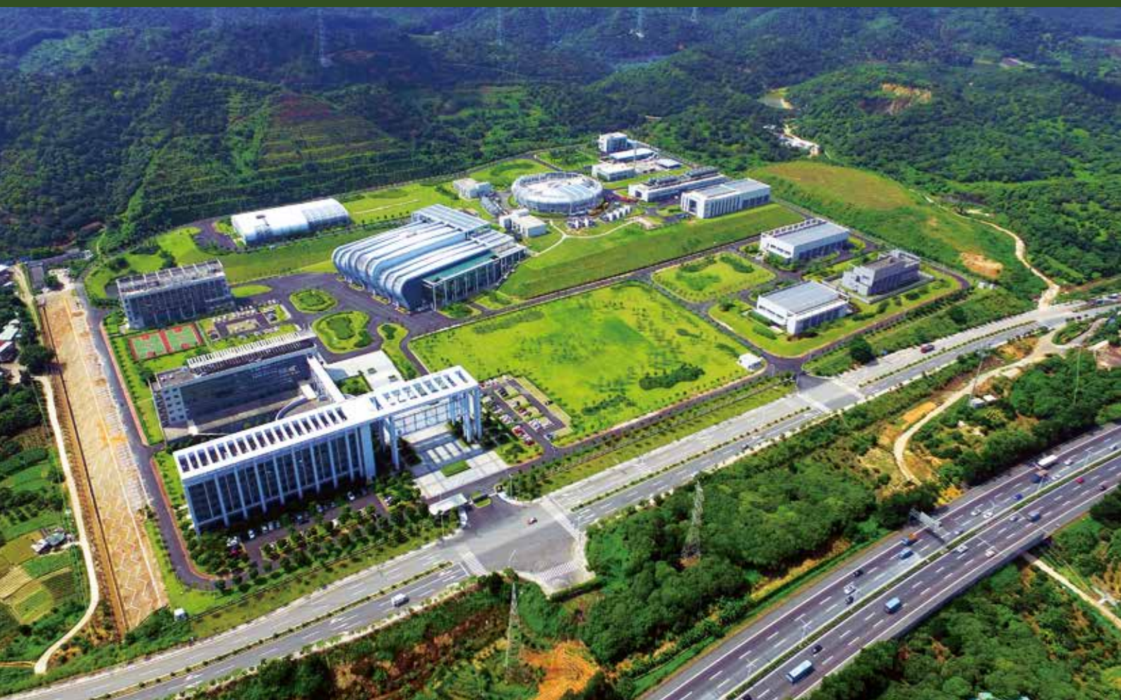
The newly completed China Spallation Neutron Source, or CSNS, in Dongguan, Guangdong Province. Credit: IHEP.
