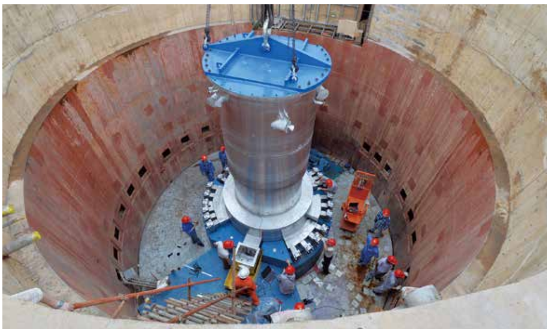
Installation of one of the helium containers at the CSNS construction site on May 5, 2015. Credit: IHEP.
