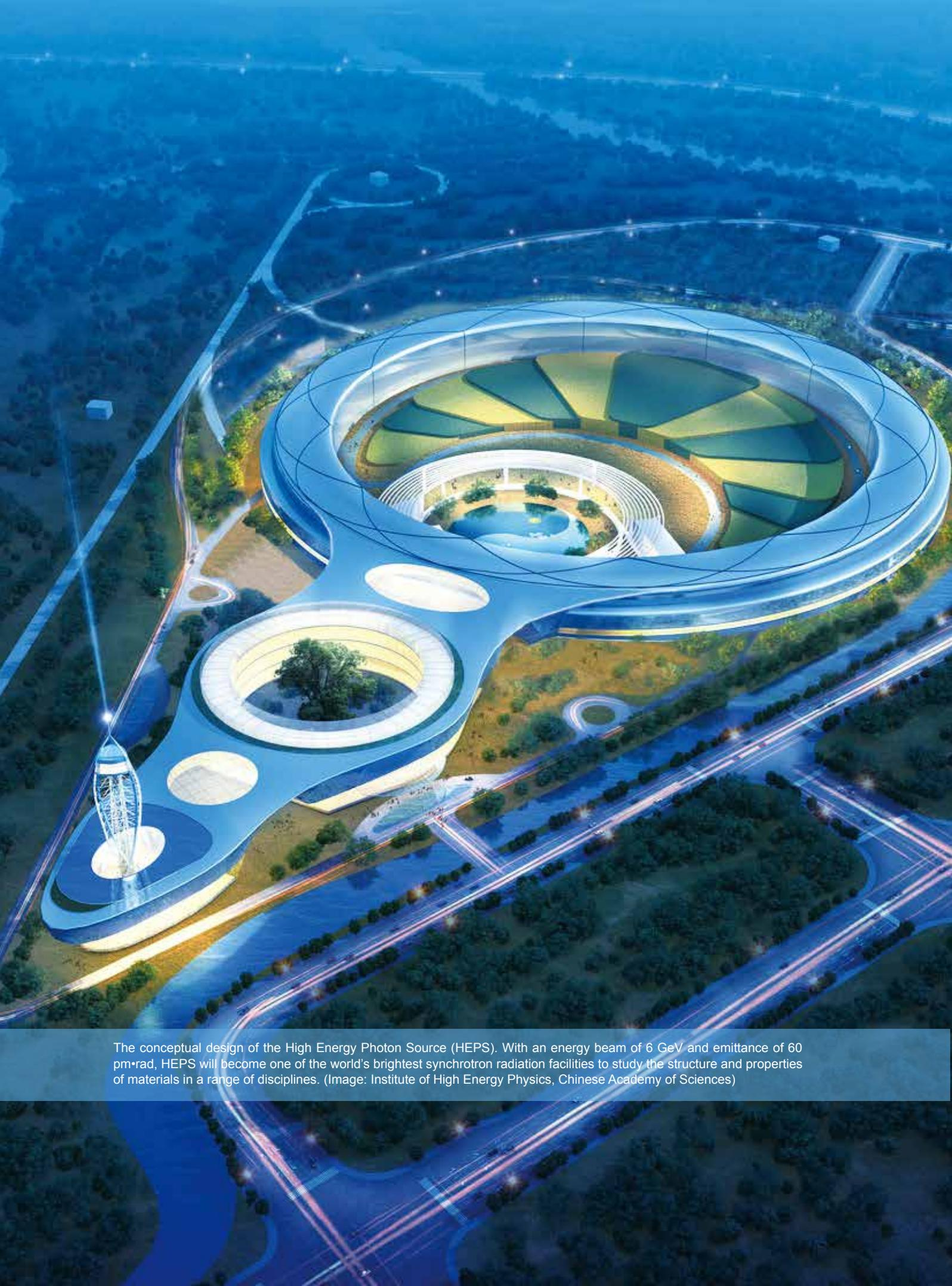
The conceptual design of the High Energy Photon Source (HEPS). With an energy beam of 6 GeV and emittance of 60 pm·rad, HEPS will become one of the world's brightest synchrotron radiation facilities to study the structure and properties of materials in a range of disciplines. (Image: Institute of High Energy Physics, Chinese Academy of Sciences)
