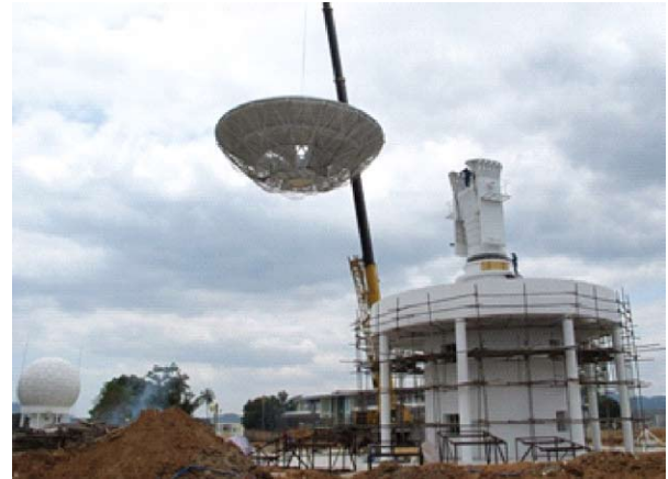
Installation of the second antenna set at Sanya Station.
