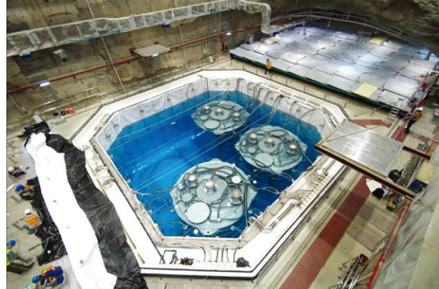
The installation of the three anti-neutrino detectors in a water pool in the Far Hall (EH3), which started taking data on Dec. 24, 2011.
