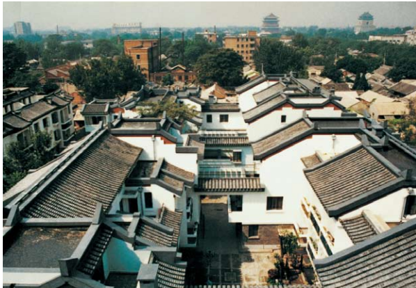
New siheyuans for an old hutong: the rehabilitation project of Ju'er hutong in inner Beijing city was completed in 1989 and won world recognition.
