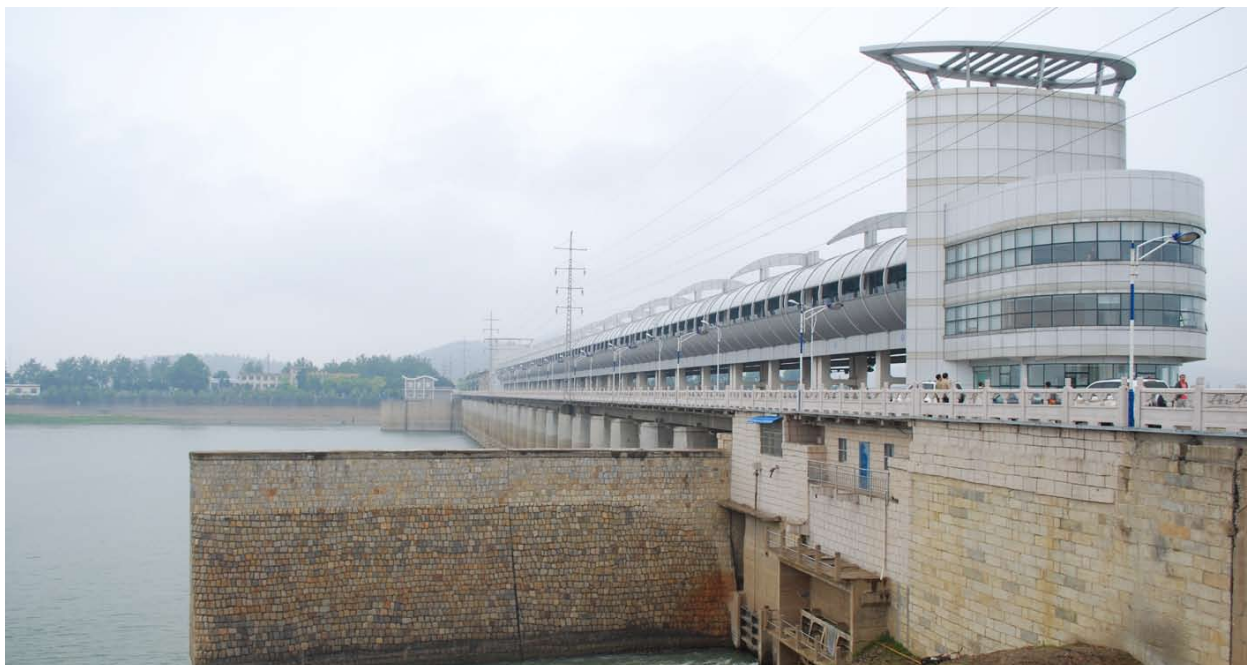
The Bengbu Sluice down the Huai River.
