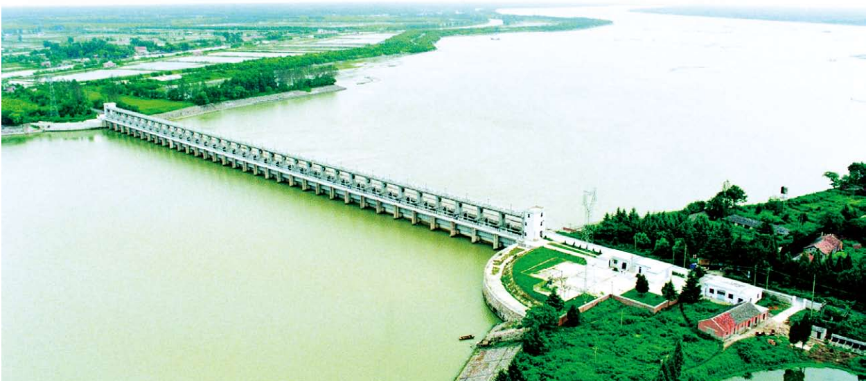
A sluice across the Huai River.
